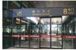
Shenyang Taoxian International Airport
