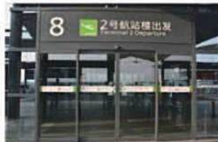
Shanghai Hongqiao International Airport
